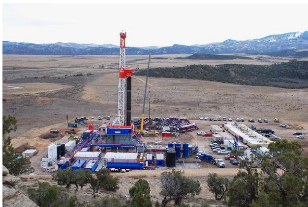
Drilling for natural gas in Colorado's Piceance Basin.
