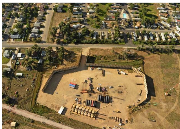
Oil and gas development in Colorado’s Denver-Julesburg Basin in proximity to a residential area.
